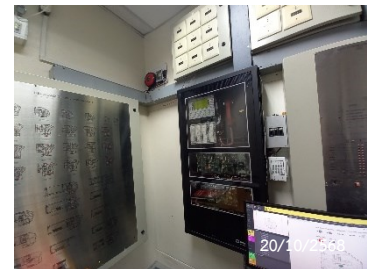
Graphic Annunciator Fire Alarm System
