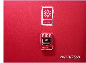
Fire Alarm Manual Station
